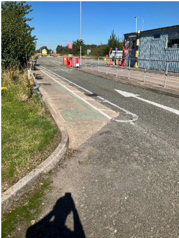
Figure 4.5 | Tata Steel Gate House Exit Lane
