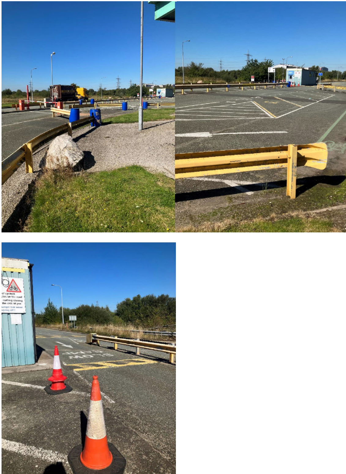
Figure 4.6 | Tata Steel Gate House Exit Lane
